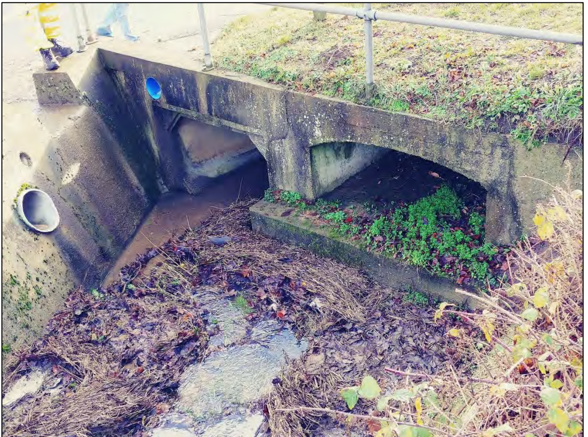
Figure 4-7 - Culvert inlet at Church Walk
