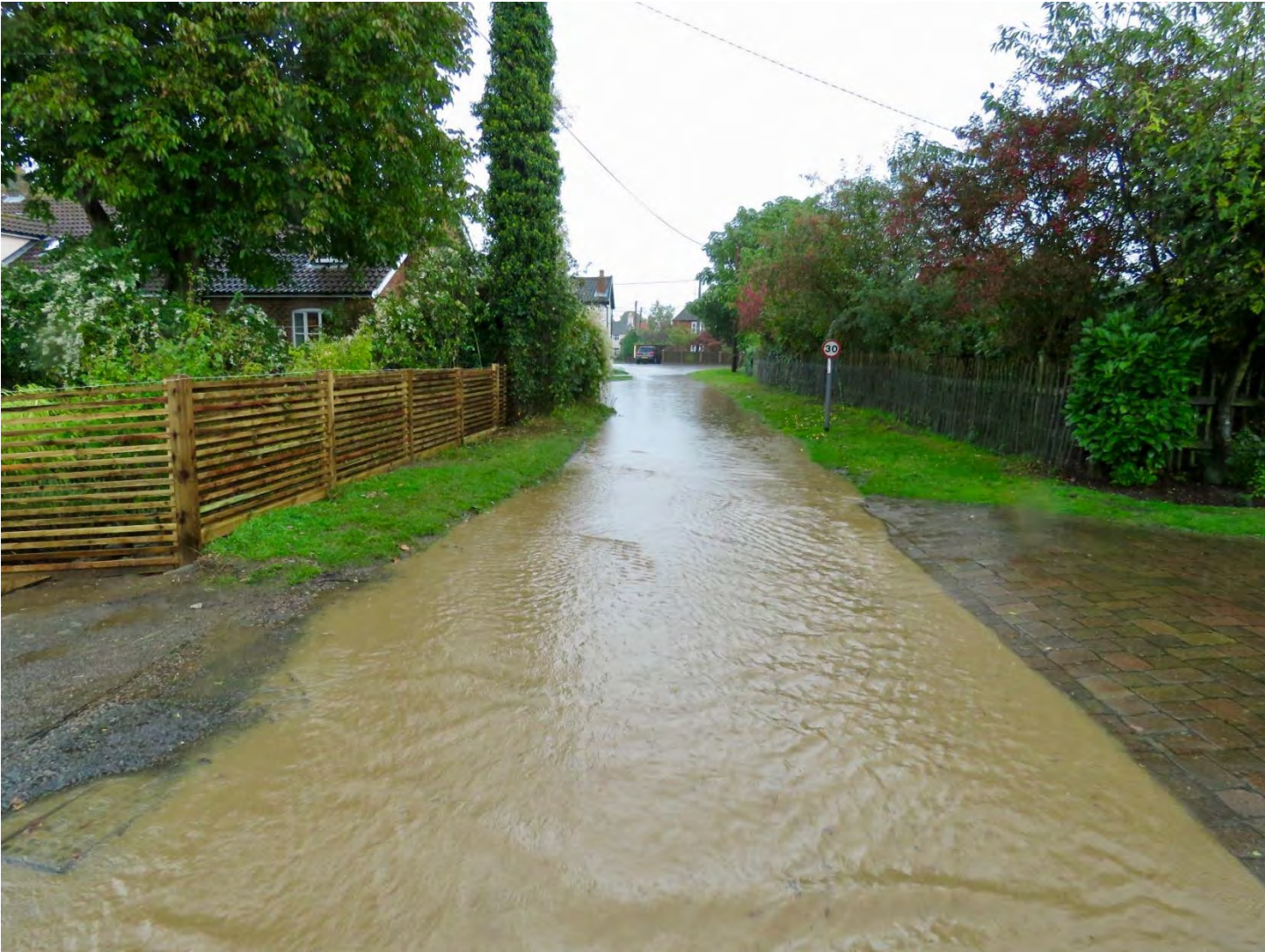
Low Road looking north towards junction with B1121
