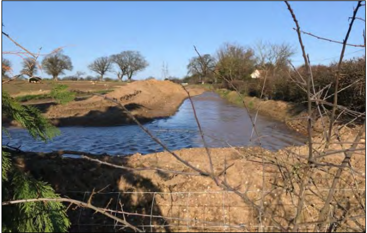
Figure 3-5 - Site visit Photograph of Pig Farm Bund and Basin
