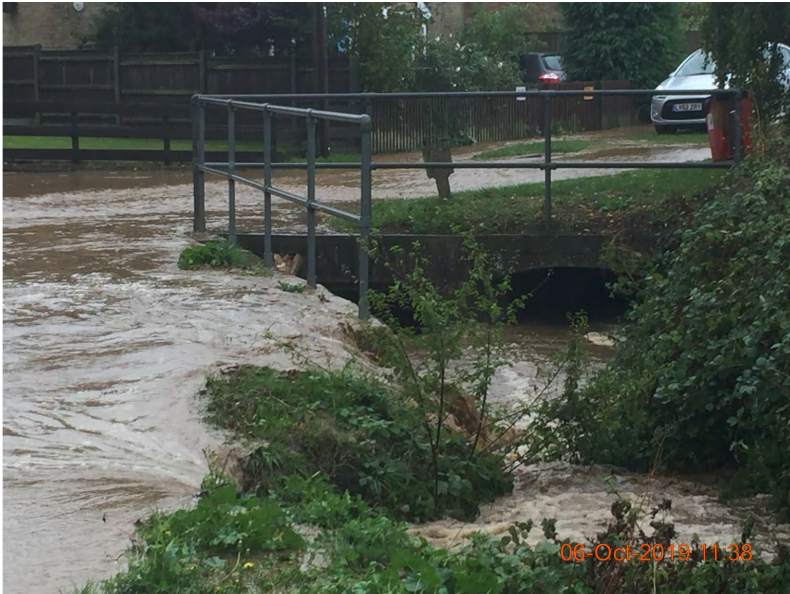
On Church Path, looking downstream to where Main River enters culvert under Friston crossroads
