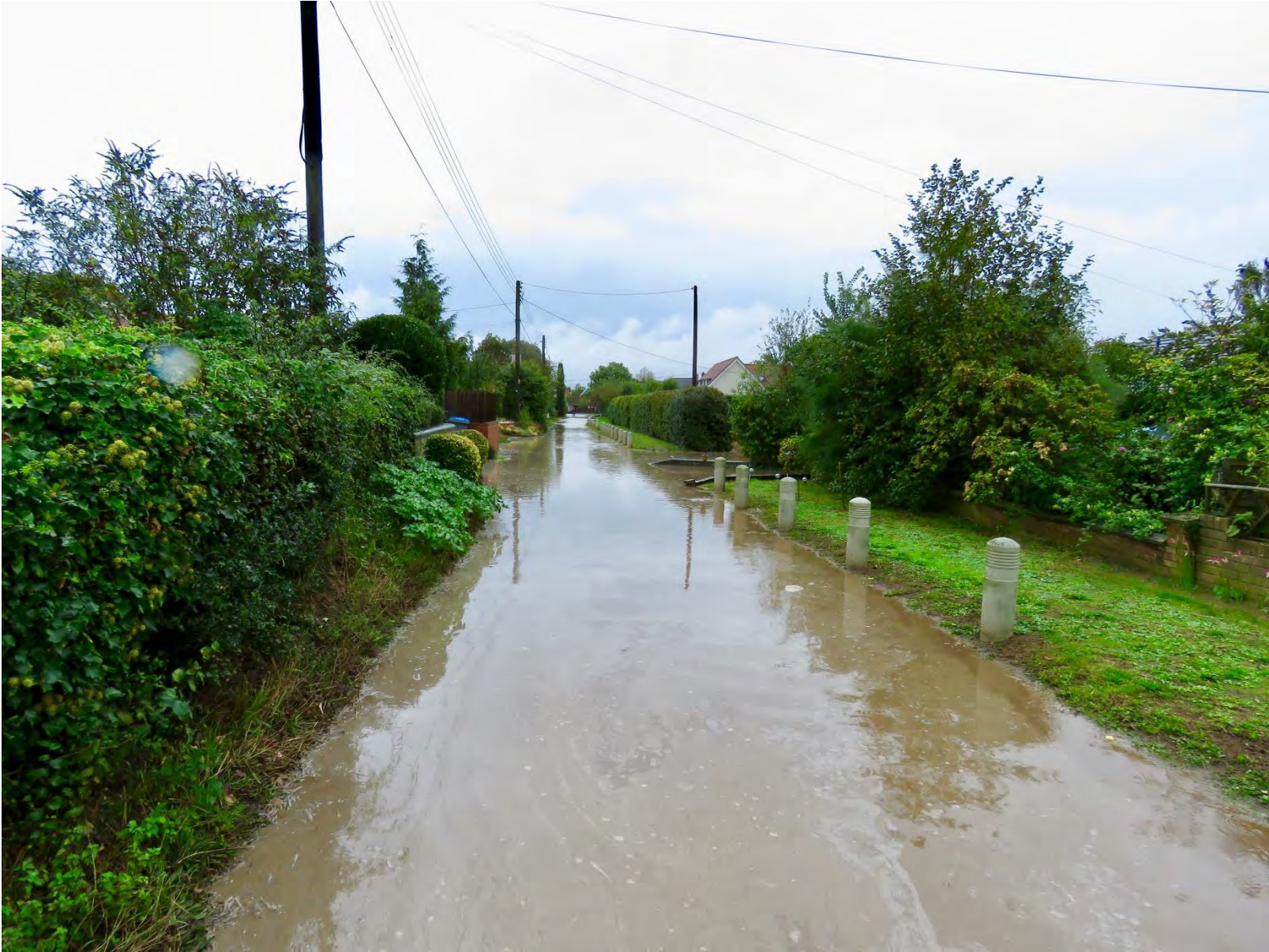
Low Road looking north towards junction with B1121 (2)
