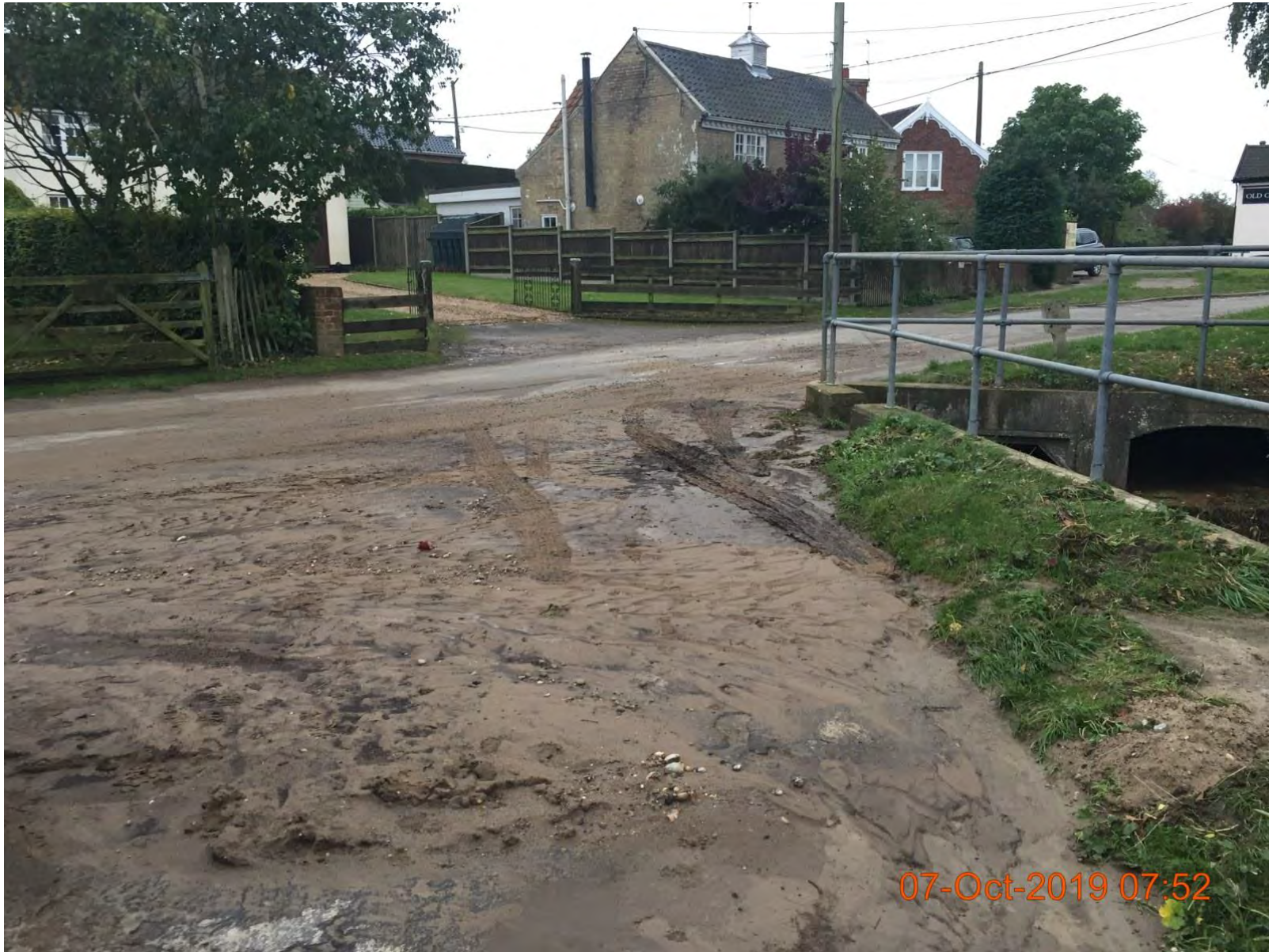
Post flood debris at Church Path
